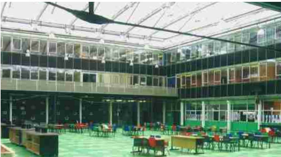
Kingsdale School in London, England, was grossly-inefficient until an architectural overhaul added a plastic-based roof for thermal insulation.
